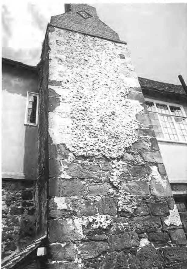
Ford Place, Wrotham: Stone stack, dated 1589, pargetted to resemble stone quoins and flint walling
