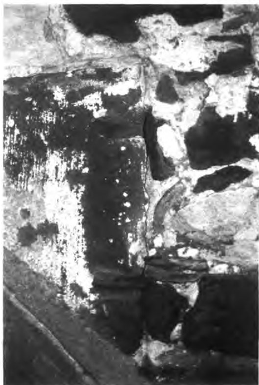
Ford Place, Wrotham: Jamb of Window seat
